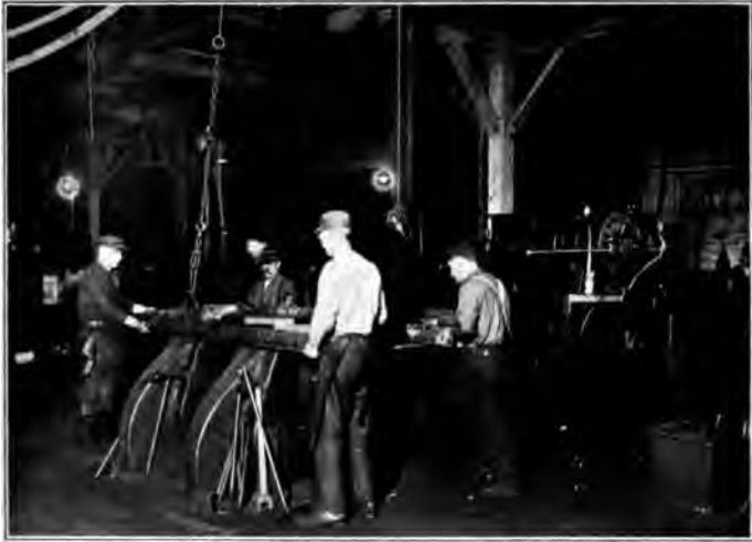
The frame end posts for Pullman standard cars are made in this section of the shops
